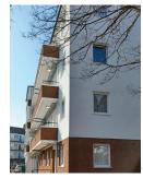
Cornerstone completed our element of the works in 2022, having worked on the nine blocks concurrently at the peak of the scheme. The EWI was applied to walls, balconies, walkways and external staircases across the three and four storeys buildings, with the mixture of textured render and brick-slips achieving a clean
